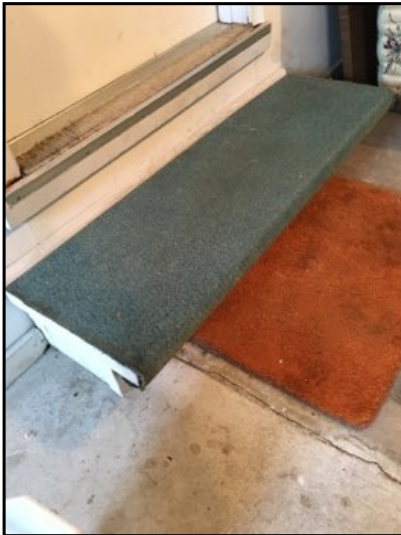
Step is unstable leading from garage to interior
